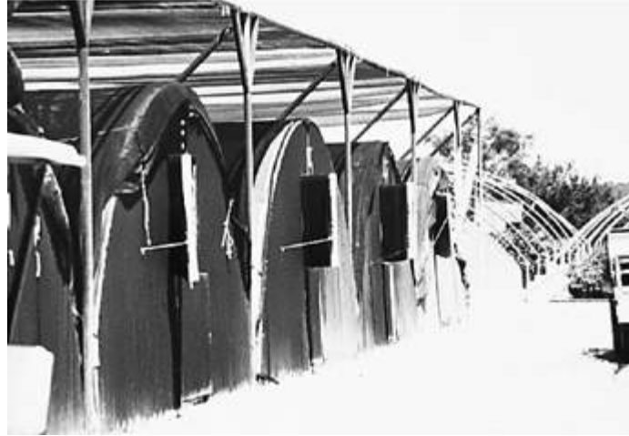
A Texas Reishi production facility. With modified hoop-framed greenhouses covered with an open-sided, metal roofed super-structure, growing rooms could be constructed at low cost.
