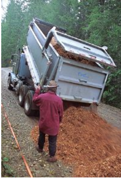
FIGURE 90 Wood chips are dumped on the road surface.
