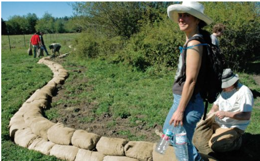
FIGURE I To reduce coliform bacteria from an upland farm, two rows of woodchip-filled burlap sacks, inoculated with oyster mushroom
